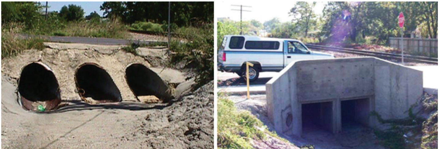
Figure 1. Old (left) and new (right) Walker Bridge
