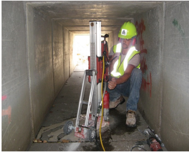
Figure 2. Sample extraction from box culvert units
